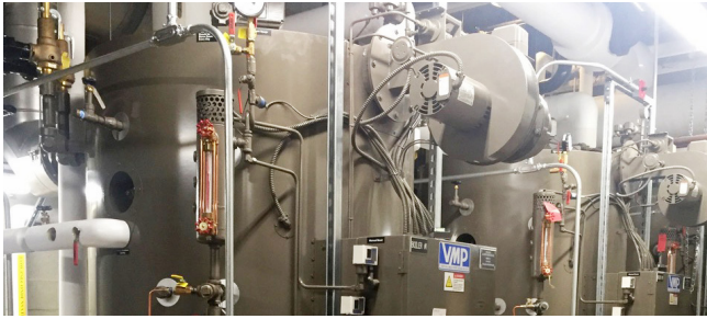
Modulating Boilers
