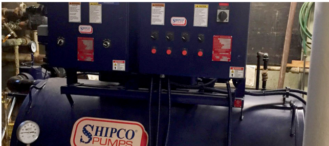
Condensation Receiver Tank
